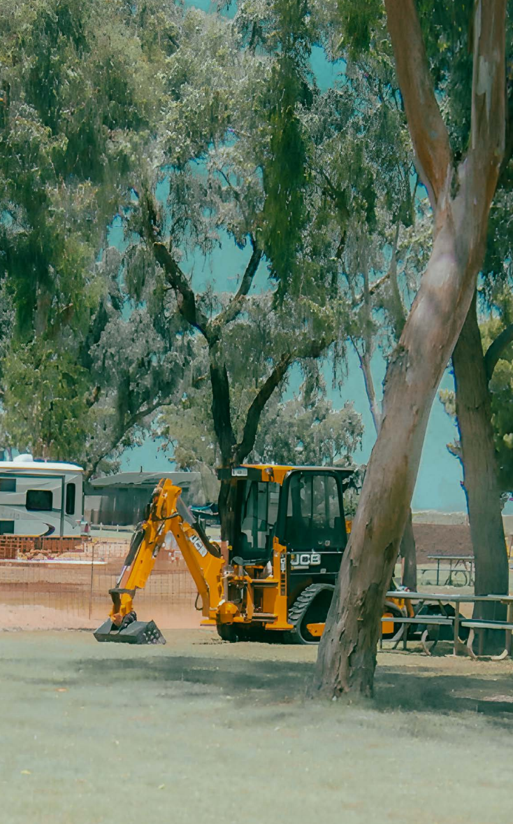
Mayflower sewer project
