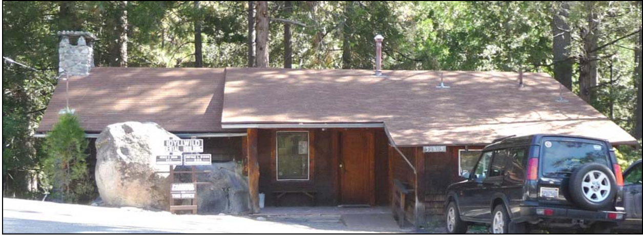
Figure 44: Incorporation of natural features (boulder)
