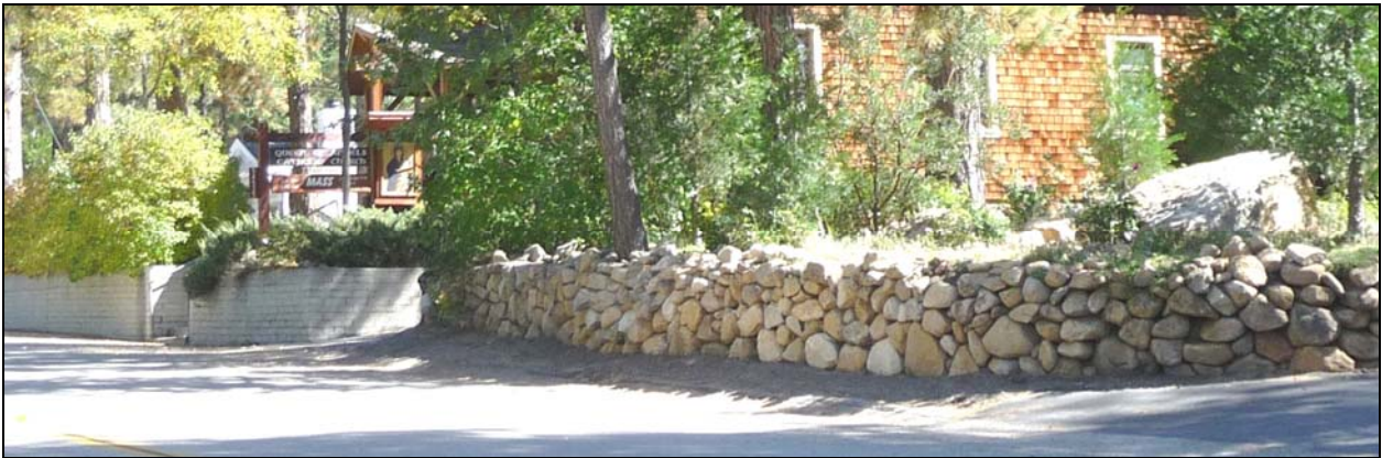
Figure 28: Two types of walls: concrete and rock
